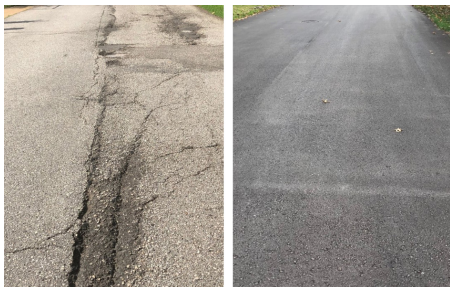
General Grant Lane - Before & After Mill and Overlay
